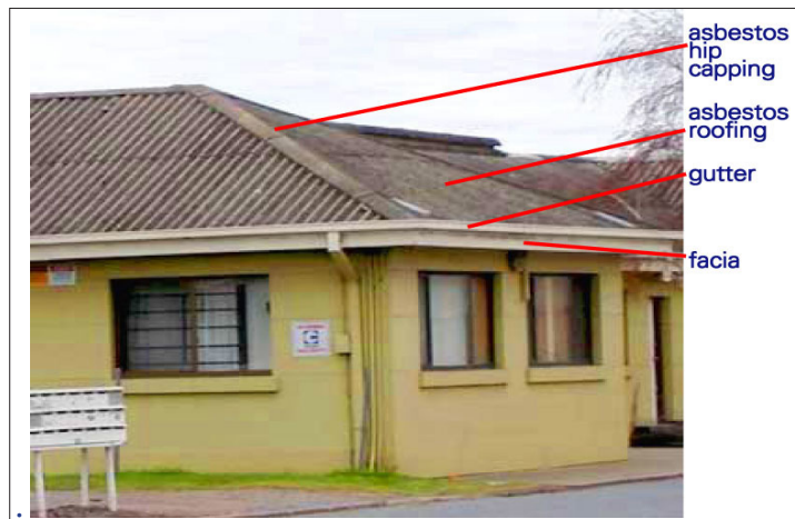
A house with asbestos roofing material.
